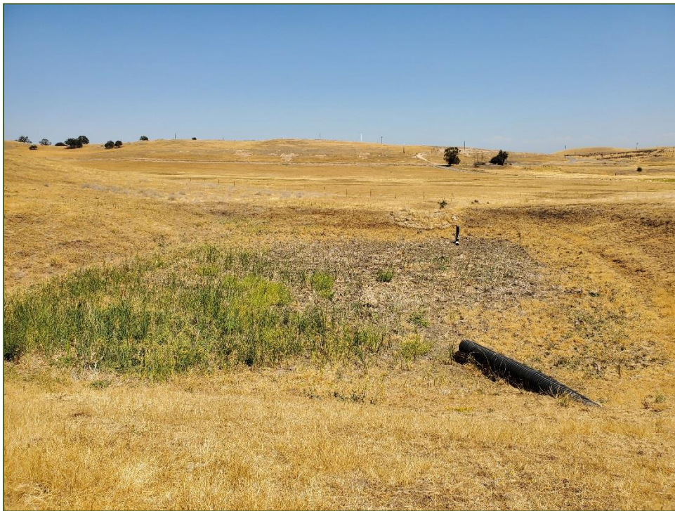
Photo 14. Basin 7 which is a earthen water quality basin constructed when the golf course was built. It is fed by the subsurface drainage system. Facing north. July 27, 2020.
