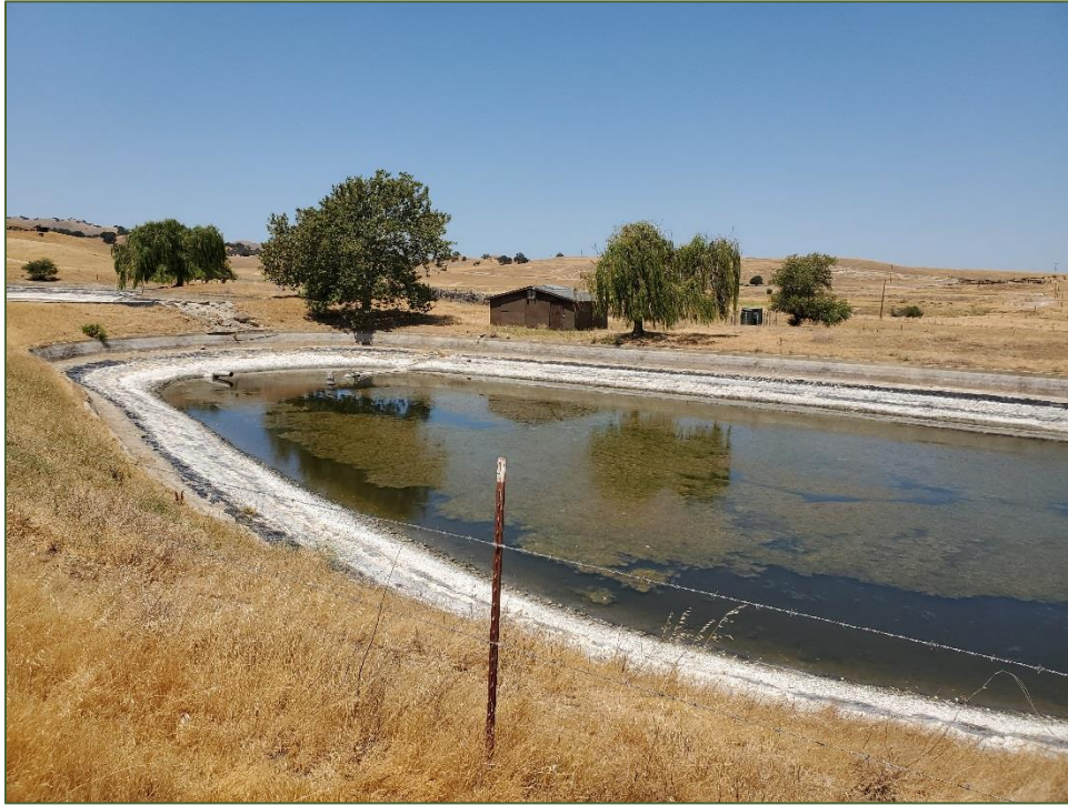
Photo 9. View of depnd031 which is a constructed concrete-edged and plastic-lined irrigation pond. The spillway from depnd030 is visible to the left of the photo. Facing northwest. May 5, 2020.
