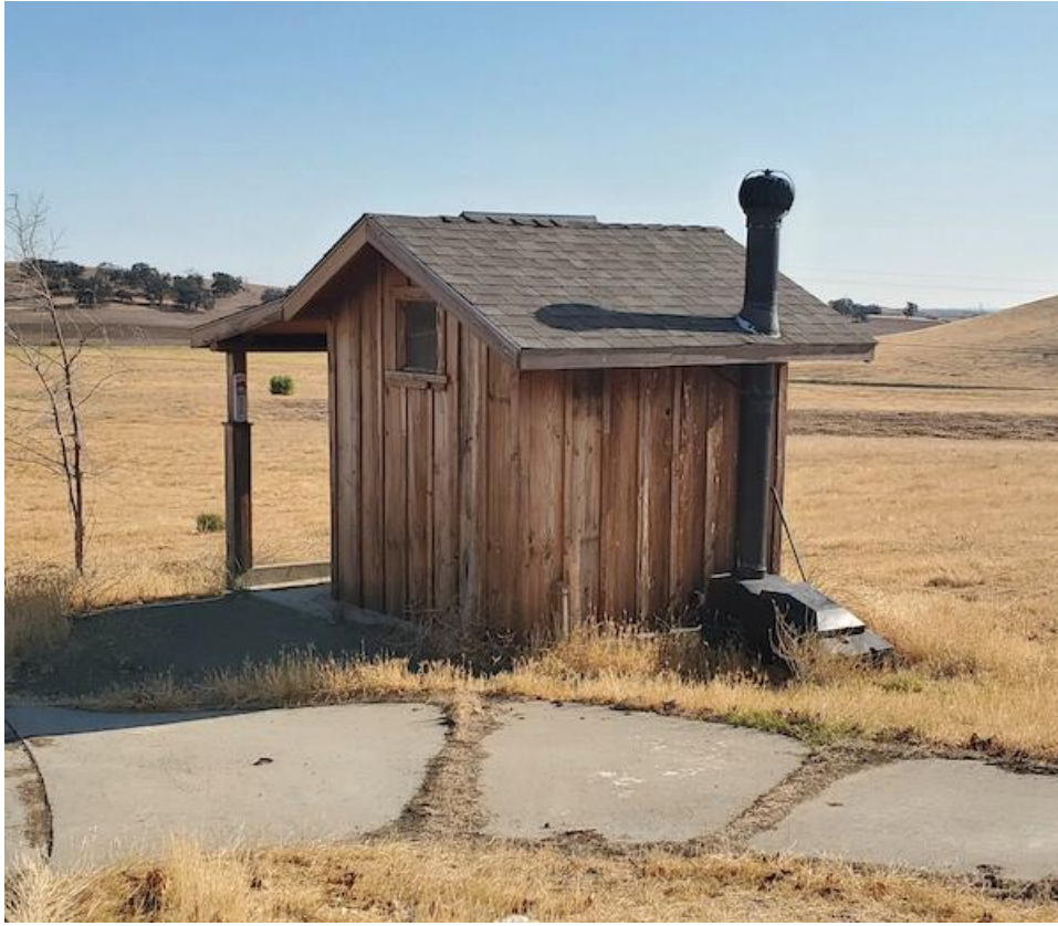
Photo 19. Restroom structure providing marginal roosting habitat for bats. Facing northeast. July 16, 2020.
