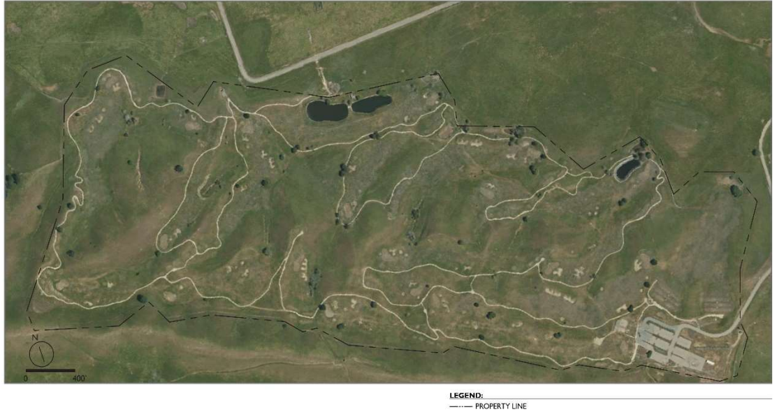
Figure 1: 2018 Aerial Photograph of the Former Roddy Ranch Golf Course
