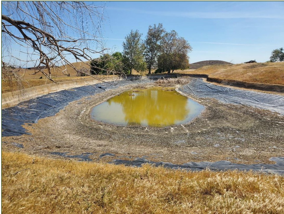
Photo 10. View of depnd032 which was a constructed concrete-edged and plastic-lined irrigation pond. A small patch of cattails was present. Facing east. February 4, 2020.
