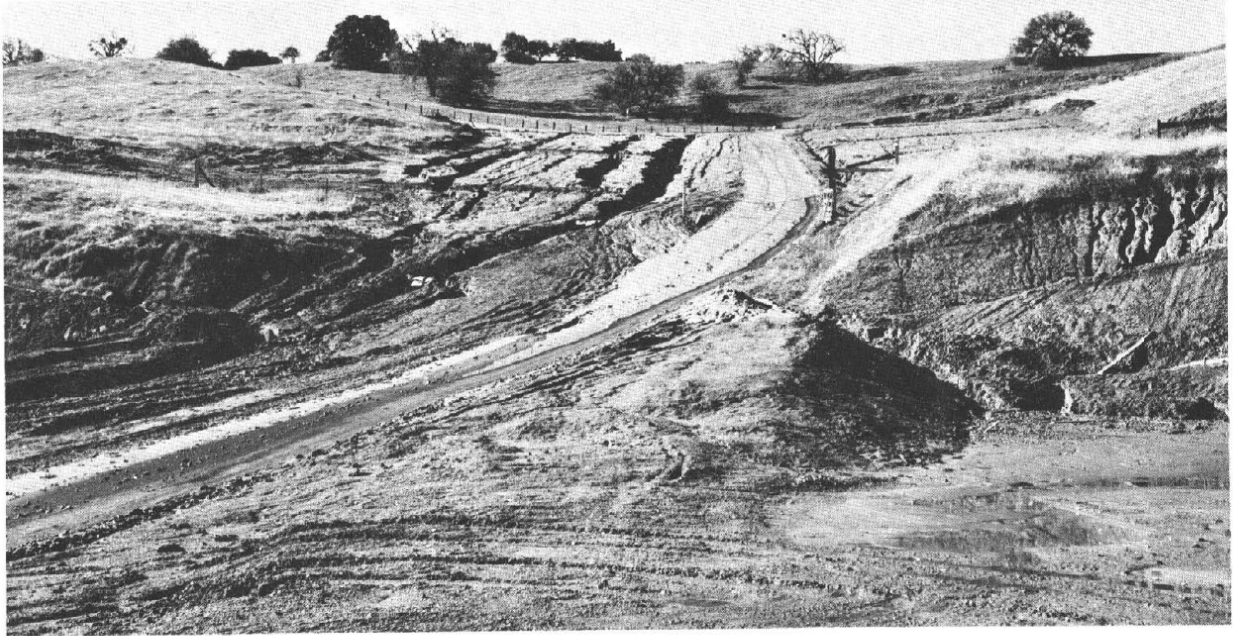
Figure 3.—Erosion in this area of unprotected Briones soils during construction contributes to sedimentation of the streams and reservoir downslope.
