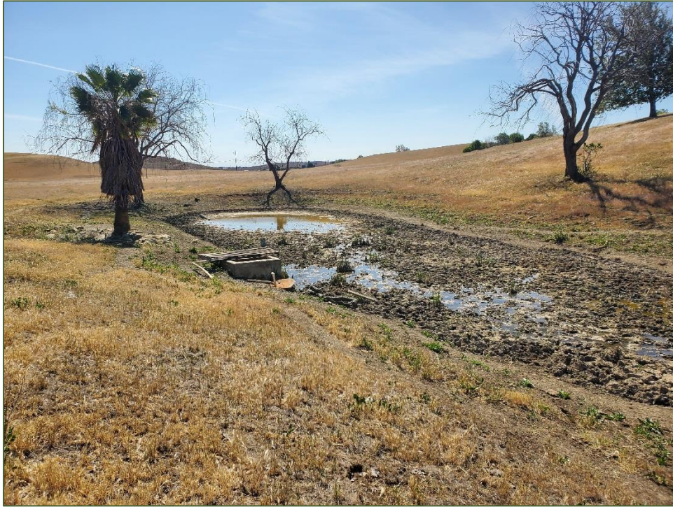
Photo 13. Basin 5 which is a earthen water quality basin constructed when the golf course was built. It is fed by a culvert from depnd031. Facing southeast. May 5, 2020.
